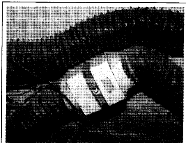
Fig. 5 Typical blower and duct system to vent fumes from the engine compartment
